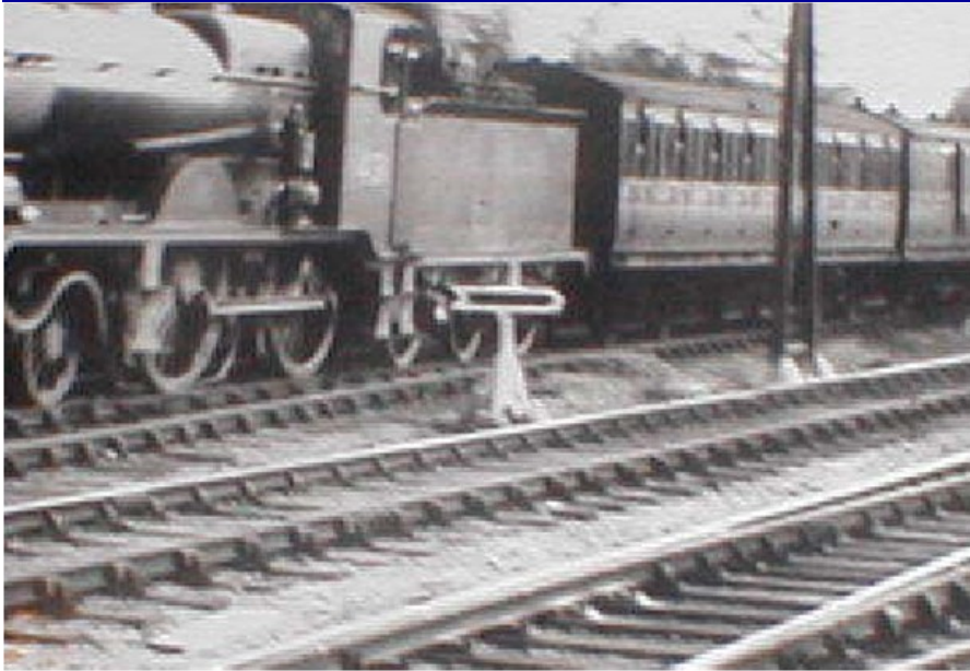
Temporary speed restriction, Croydon
