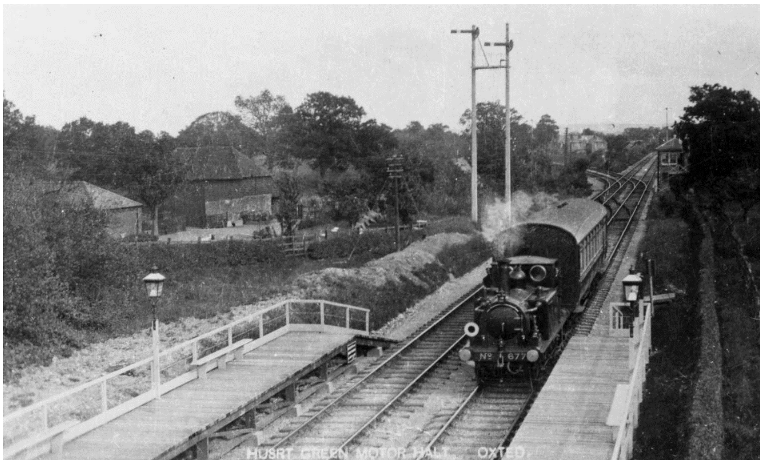
Hurst Green halt – a typical timber platform with minimal facilities. Terrier 677 on autotrain.
