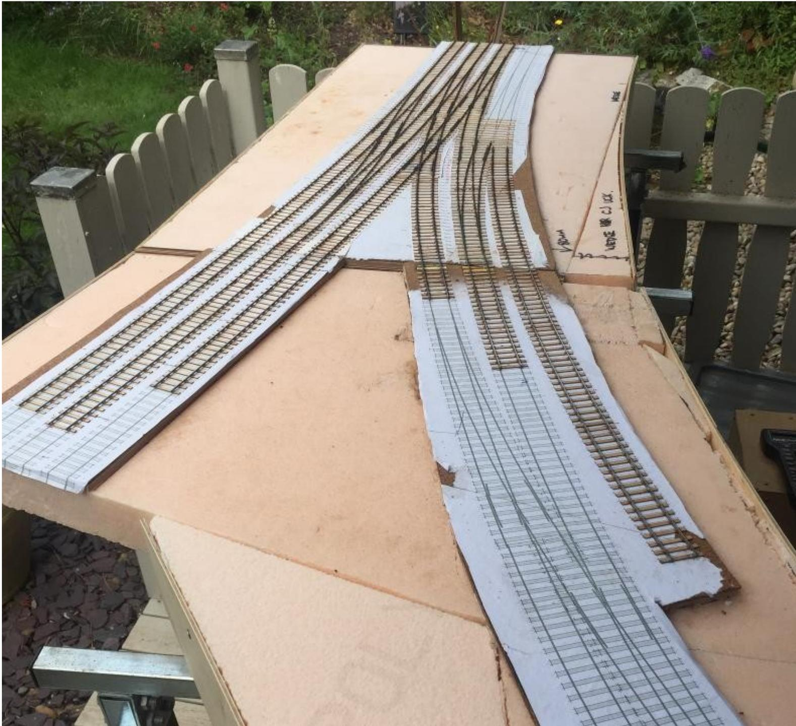
Figure 10 The completed 'country junction' with some plain line added, including across to the next board for the station junction.
