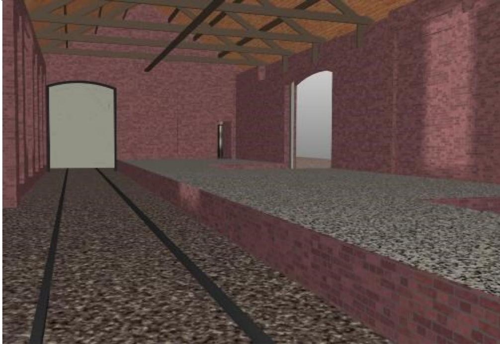
I don't usually model the interiors of the building but, having a good photograph to work with, I have included some of the structural roof detail. I was also intrigued by the loading bay doors and how they opened. The wall structure and step back above the doors all indicate that the doors slide into the wall. I have not seen this before so would be interested in comments regarding this.
